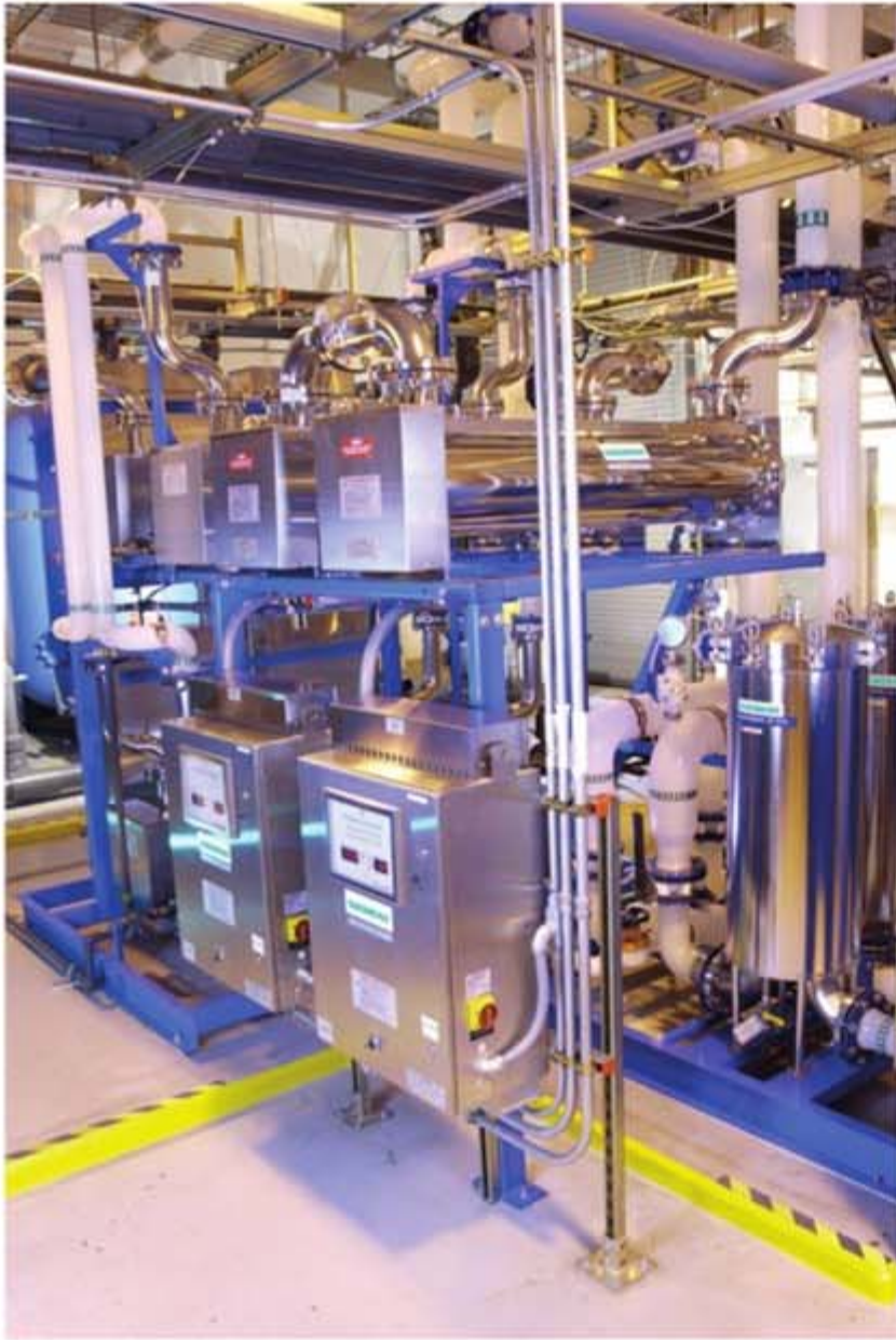
Figure 2. A typical UPW UV system.
