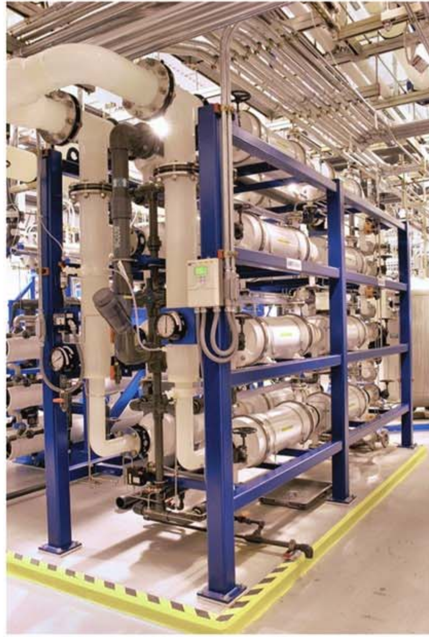
Figure 3. A typical UPW membrane degasification system.
