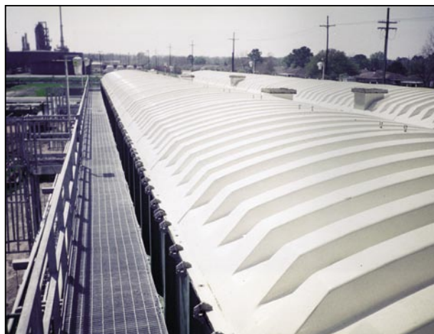
FIGURE 7. To prevent emissions of volatile organic compounds, many API separators are outfitted with covers
