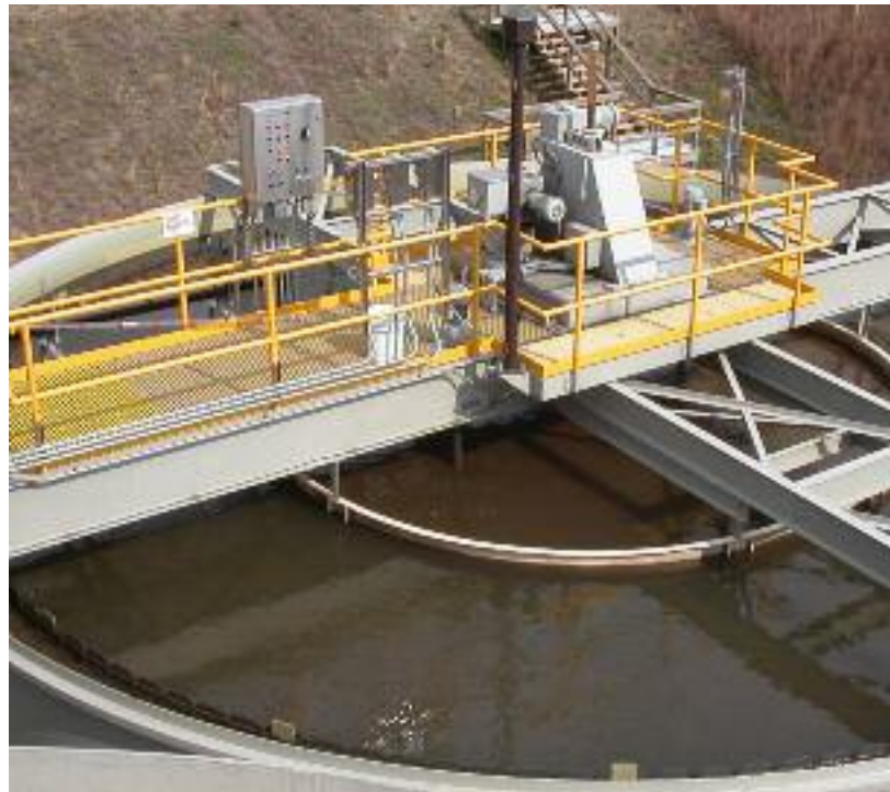
We provide a wide variety of clarifiers to treat surface water for suspended solids, hardness and turbidity removal.
