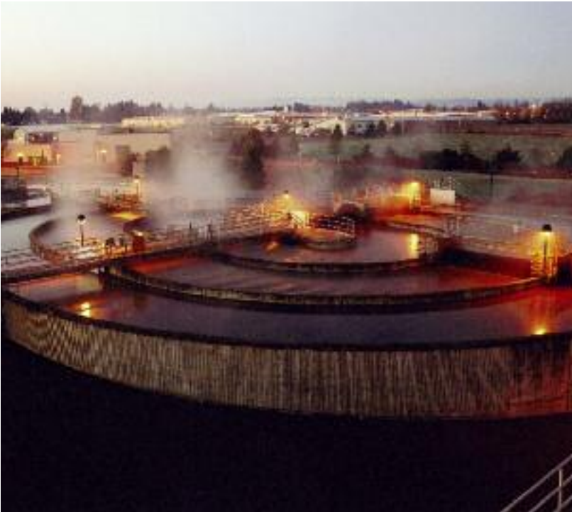
The Orbal® aeration system has been proven for performance and flexibility of total nitrogen control in numerous petroleum applications.
