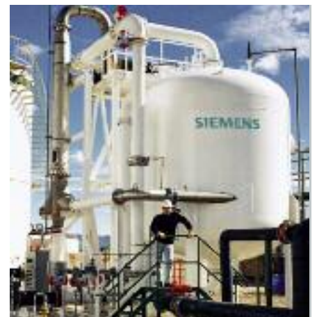
Walnut shell filters remove almost 100 percent of free oil from produced water.
