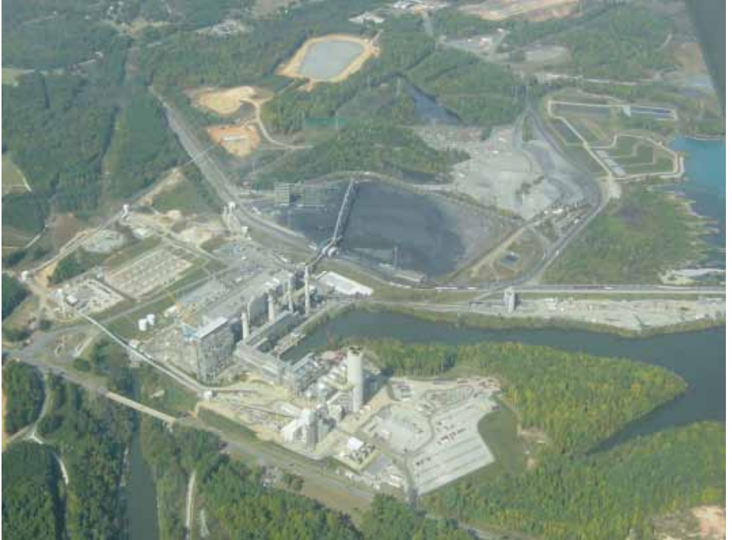
Figure 3: Marshall Station FGD System and WWSRS
