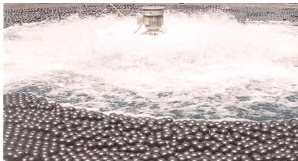
The floating balls are pushed away and stacked up by the aerator spray.
