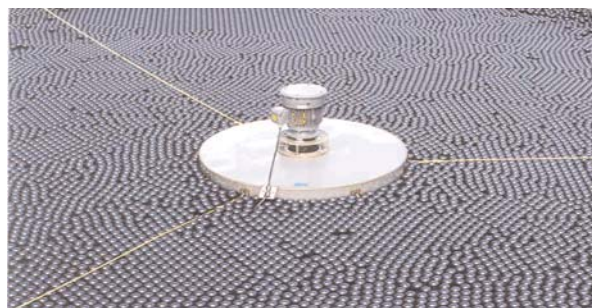
The floating balls recover to a single layer when the aerator is turned off.
