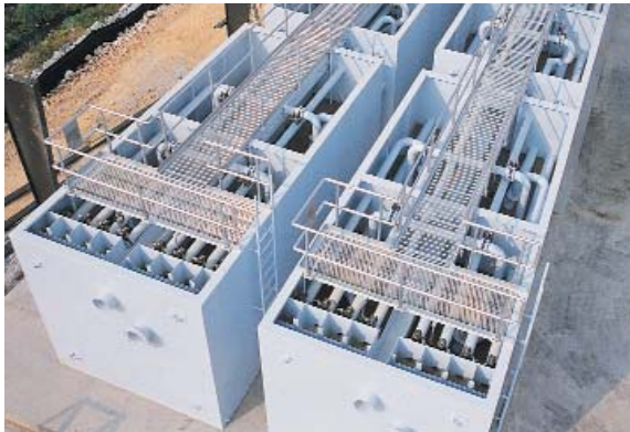
The addition of denitrification filters are perfect for existing installations required to incorporate nutrient removal due to stricter effluent regulations, without modifying or altering the existing equipment or treatment process.
