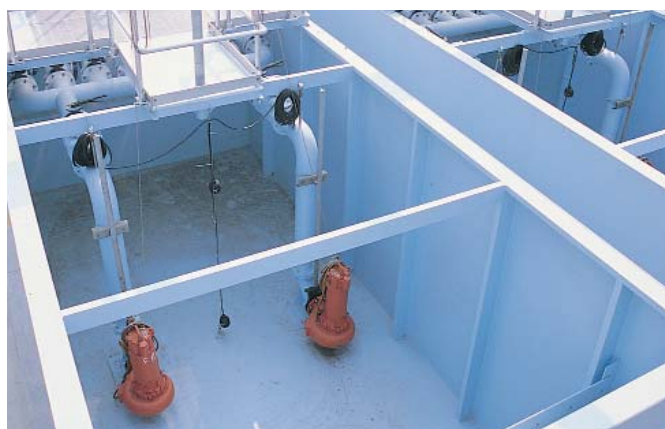
Clearwell, pumps, and control valves are included in the complete denitrification filter steel package.
