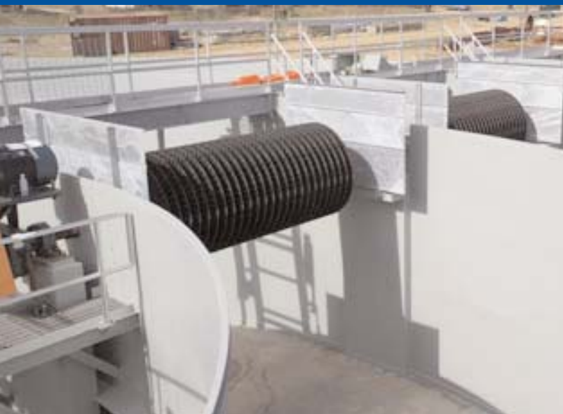
Aeration disc installed in Orbal® multichannel oxidation ditch
