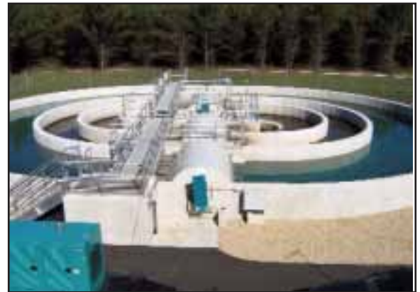
Small Flow Orbal System with Concrete Walls
