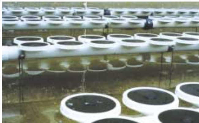
The DualAir membrane fine-bubble diffuser systems' design – two diffuser bases connected by a curved saddle that fits over conventional CPVC air distribution piping – allows twice as many saddles to be mounted to a given length of pipe, compared to conventional single-pod diffuser designs.
