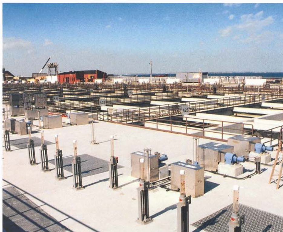
View across project to Boston Harbor.
