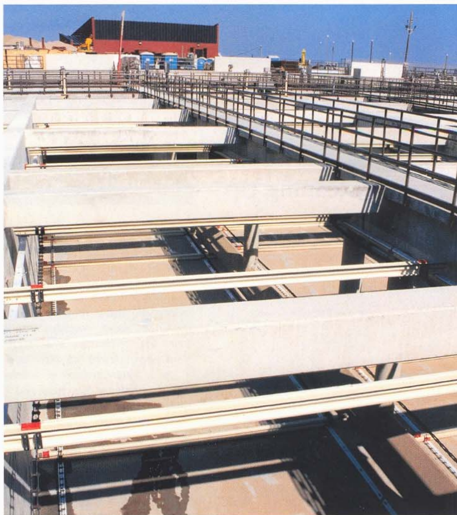
World's largest installation of chain and flight collectors.
