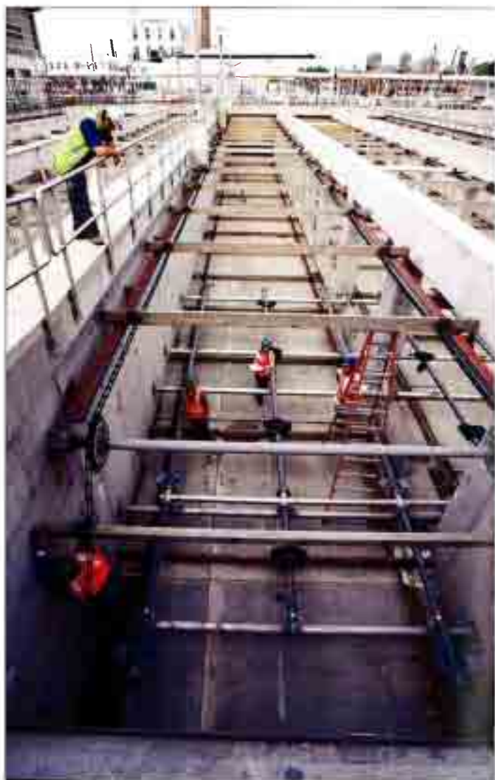
▲ Fitting Out. Solids handling equipment is placed into tanks.
