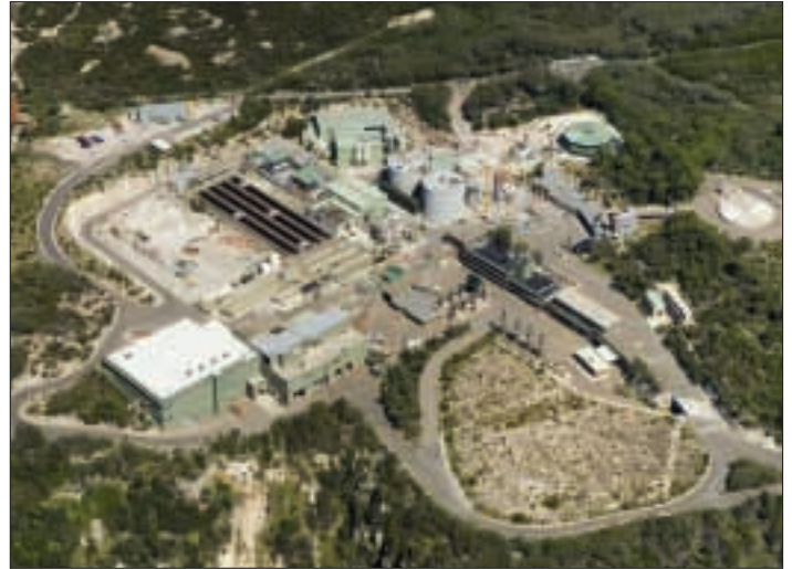
Three digesters and the gas-holder building can be seen in the upper right. Photo by SWC
