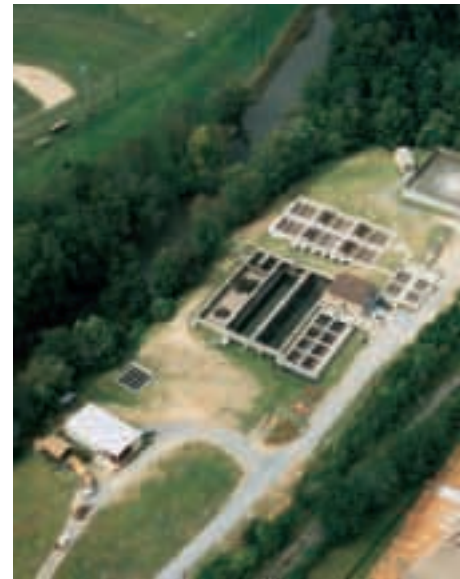
The basins of the Vertical Loop Reactor system share common walls, reducing construction costs.
