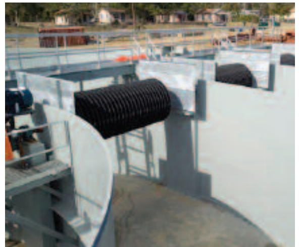
Aeration disc installed in Orbal® multichannel oxidation ditch
