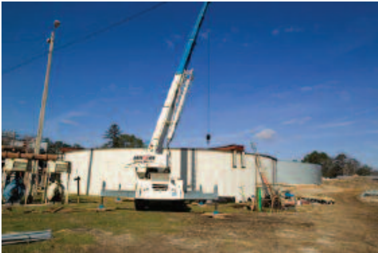
Installation of the Davco™ field-erected tanks can be easily constructed by a qualified contractor or by one of the Siemens field installation teams. Our crews are experts in the field erected treatment plant assembly methods. They have earned an exceptional reputation for quality on-site workmanship and reliability in meeting or exceeding schedule and budget goals.
