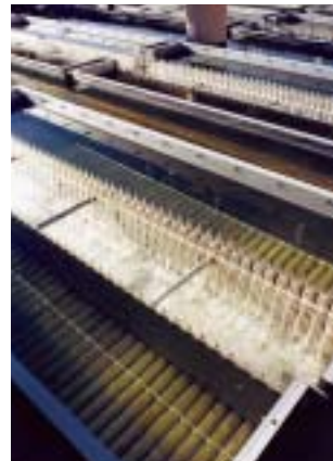
USFilter will provide 72 stainless steel plate packs for installation in four sedimentation basins at the 60 mgd Gwinnett plant.
