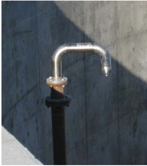
Optional top nozzle for breaking surface crust.
