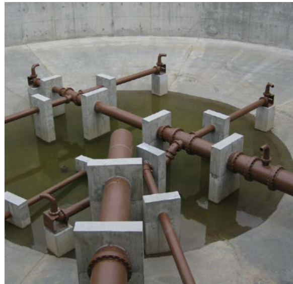
JetMix™ Vortex Mixing System arranged for optimum mixing efficiency.
