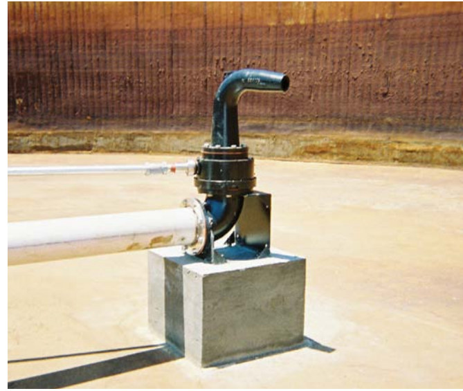
Optional rotatable mixer nozzle.
