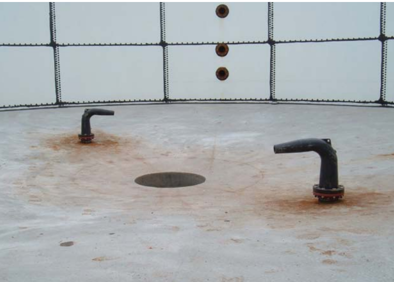
JetMix™ Vortex nozzles mounted to tank floor.
