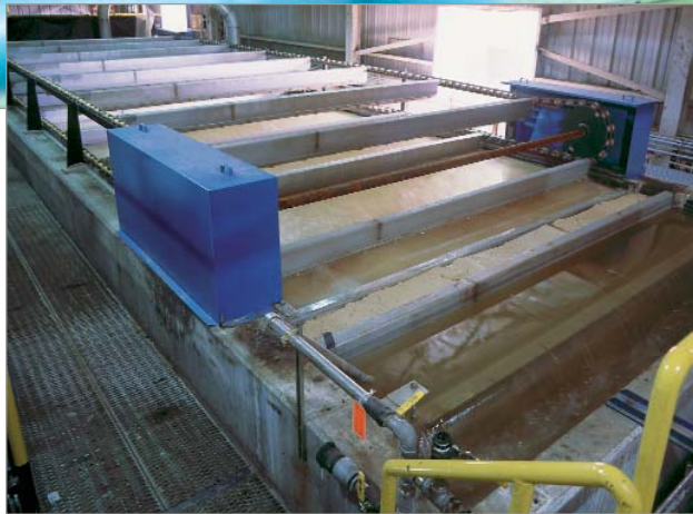
Figure 3. In DAF separators, influent is mixed with countless micron sized air bubbles as the flow enters the tank.
