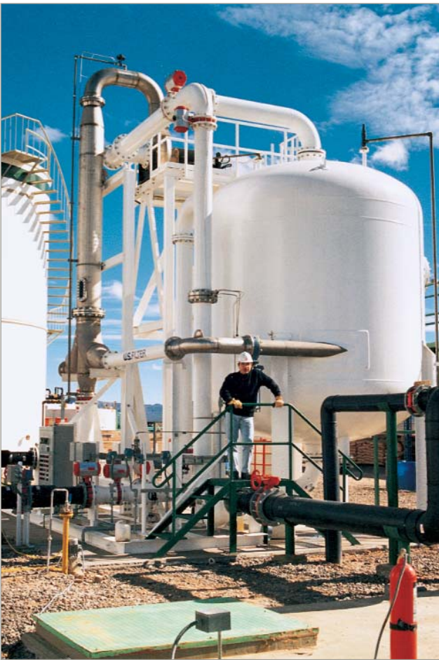
Figure 2. Tertiary produced water separation treatment methods include walnut shell, media, cartridge and activated carbon filtration.
