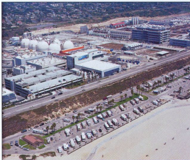
The 55-year-old facility serves some 4 million area customers and treats 340 mgd of wastewater.
