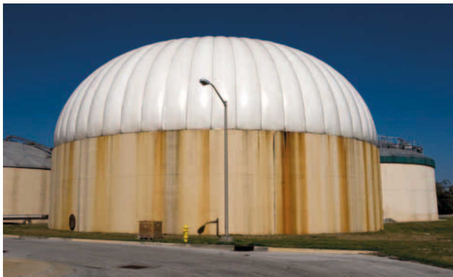
The Dystor ® system is a digester gas-holder design that uses a dome-shaped, engineered membrane system to prevent odors and store methane gas and sludge. The system includes two durable membranes. The outer membrane is cable-restrained and remains inflated in a fixed position. The inner membrane moves freely as it stores or releases gas generated from the anaerobic digestion process.
