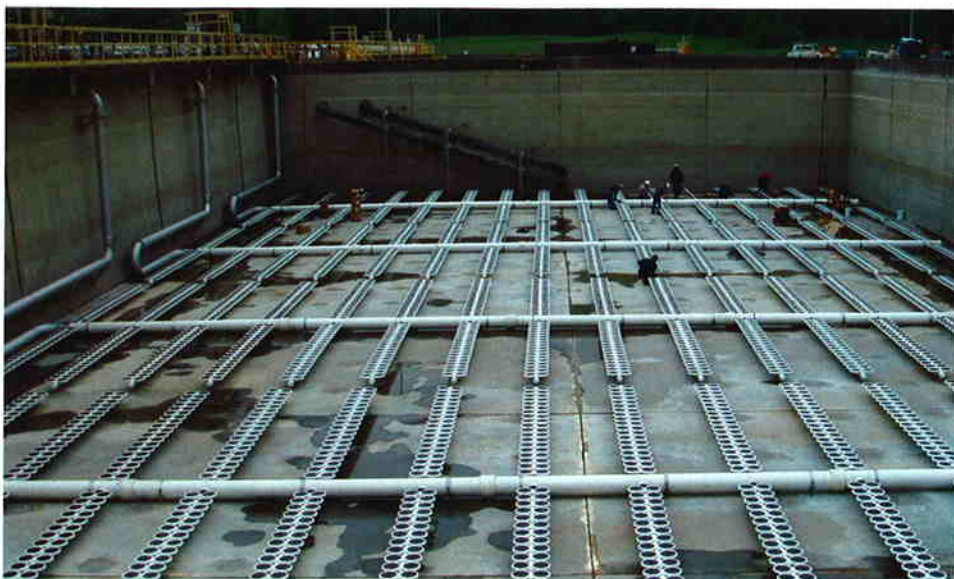
A DualAir system using cooling loops (loops are on left side of tank).
