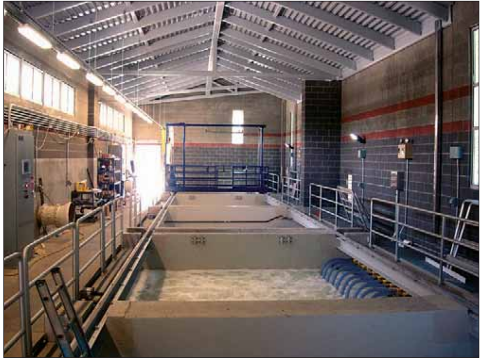
The membrane modules allow the water to be reclaimed for additional uses.
