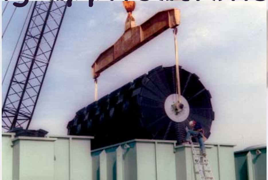
Figure 1. After installing the two air headers, the media shaft is fitted into the tanks in one pick/placement. Each unit is put into service less than 50 hours after the tanks are set.
