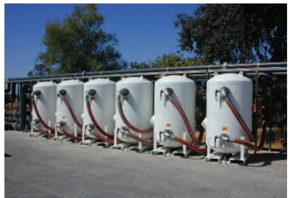
MagFlex® vessels from Siemens in a lead/lag configuration
