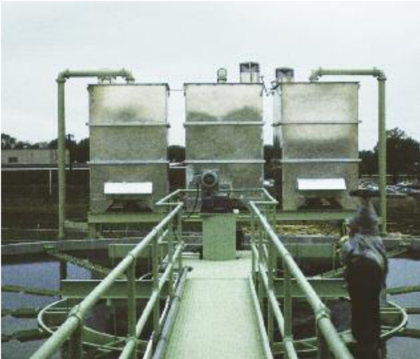
4.75 MGD Aerator Installation
