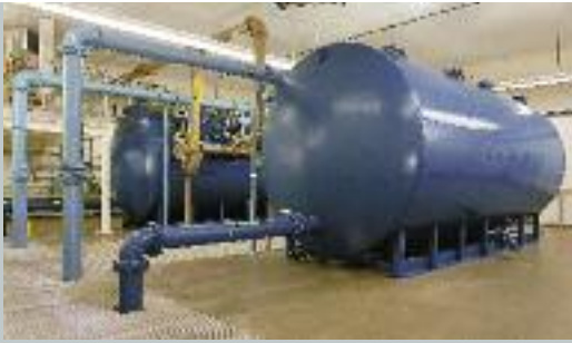
Horizontal pressure filters
