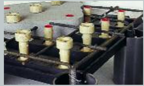
MULTICRETE II prior to concrete placement.
