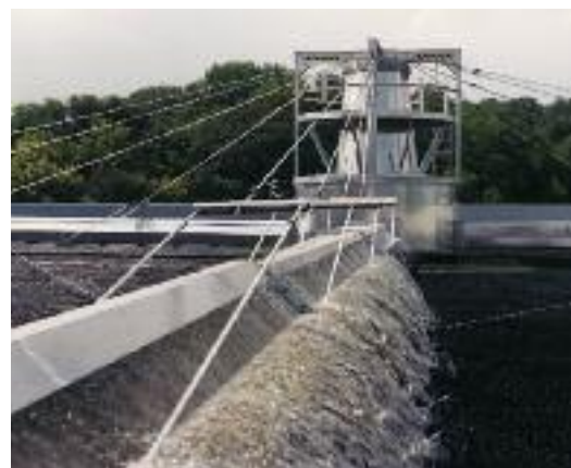
Hi-GARD arm provides even distribution of flow.
