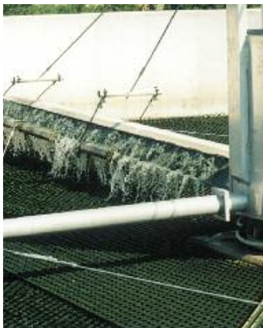
All-aluminum 50 ft. diameter, 2-arm Hi-GARD.
