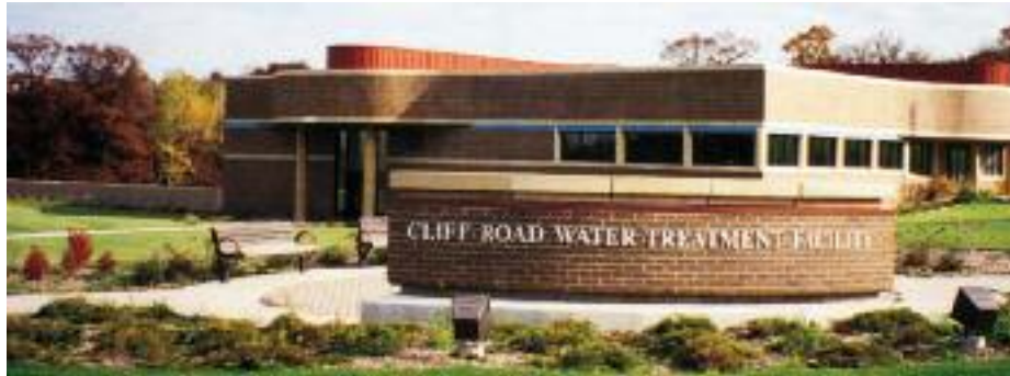
20 MGD (76 MI/d) Water Treatment Plant Utilizing MULTIWASH systems CentROL Filters
