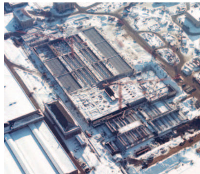
Detroit's Water Works Park II project, under construction.
