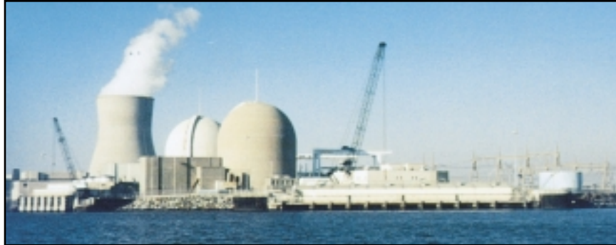
PSEG's Salem Generating Station
