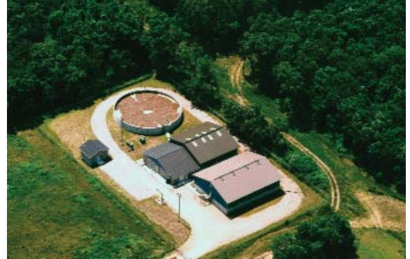
Ho-Chunk Nation Wastewater Treatment Facility
