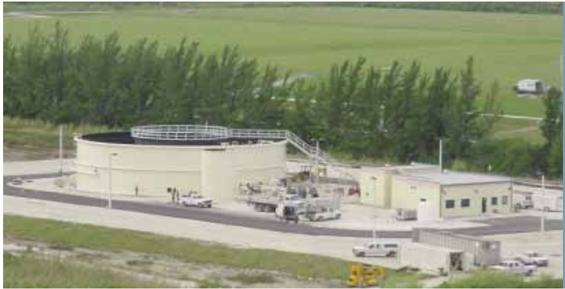
OMNIPAC® Field-Erected SBR installed at municipal wastewater treatment plant
