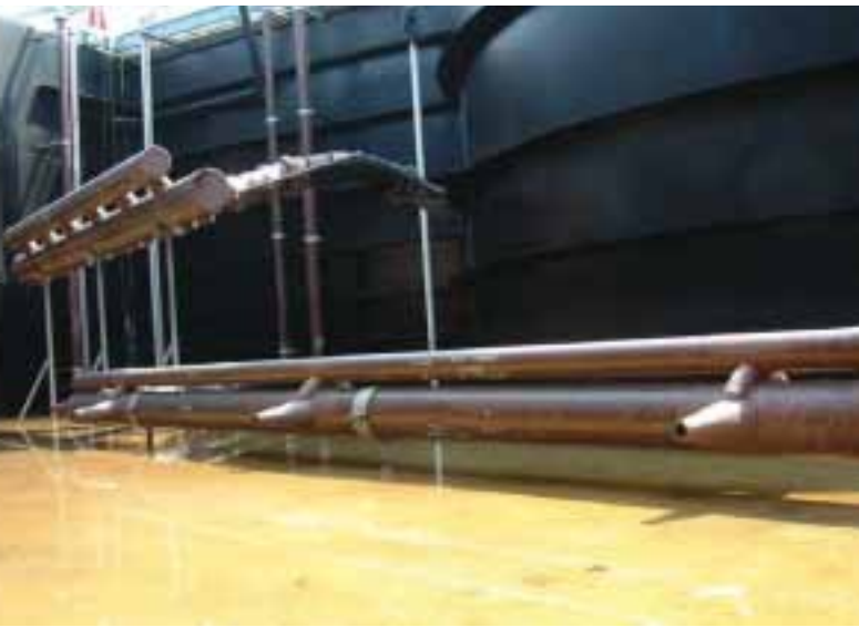
VARI-CANT® Jet Aeration System and Floating Solids Excluding Decanter installed in OMNIPAC® Field-Erected SBR
