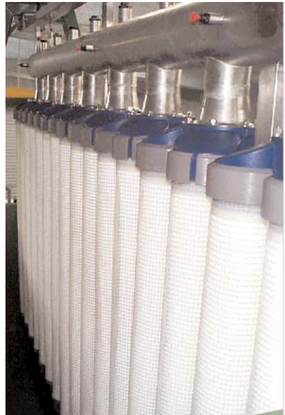
Memcor CS Module Assembly
