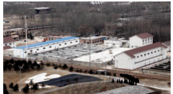
The MBR Plant
