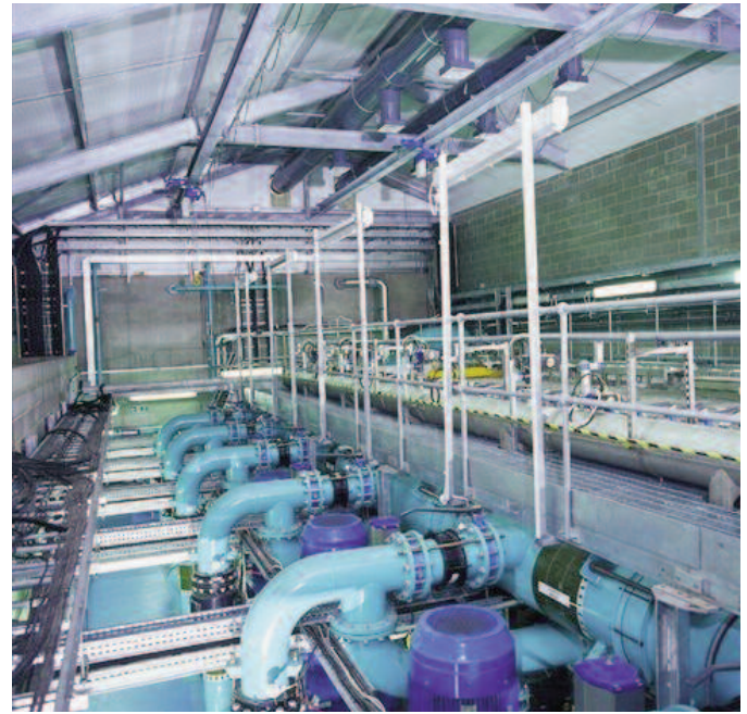
Memcor® Submerged continuous microfiltration plant provides a barrier to CRYPTOSPORIDIUM, irrespective of the feed water quality.
