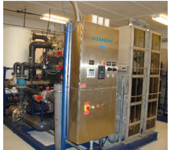
This pre-engineered skidded system is pre-wired, pre-piped and factory tested before shipment.
