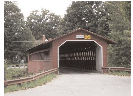
Henry Bridge over Walloomsac River
