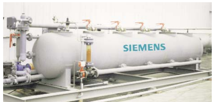
Hydrocell® separator cylindrical design.
