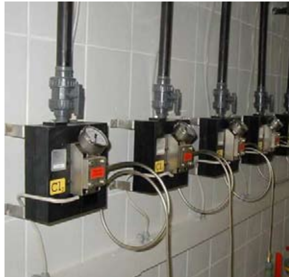
60 kg/hr (3,168ppd) vacuum regulator
