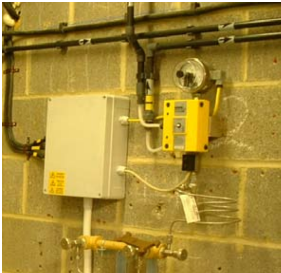
5kg/hr (264ppd) vacuum regulator
