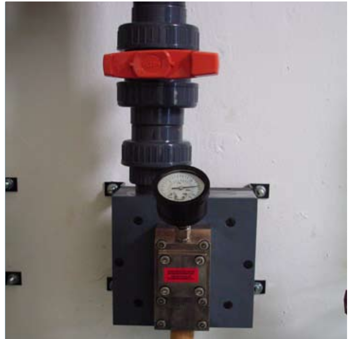
250kg/hr (13,200ppd) vacuum regulator
