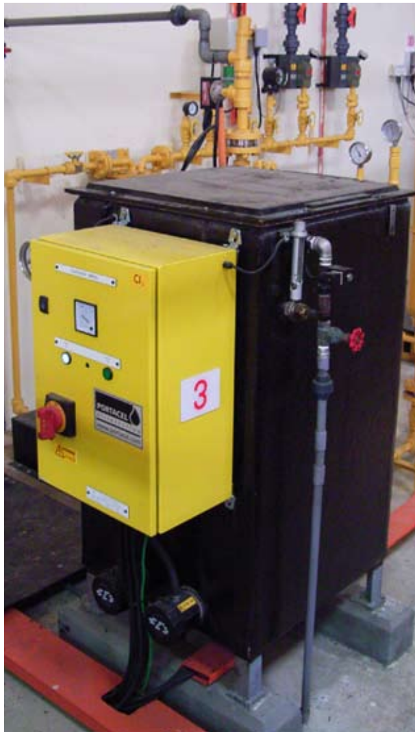
Installed Series 200E Evaporator
