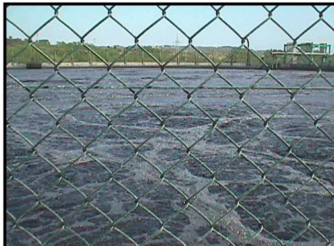
Figure 4. 65 m diameter PACT-1 aeration basin.
